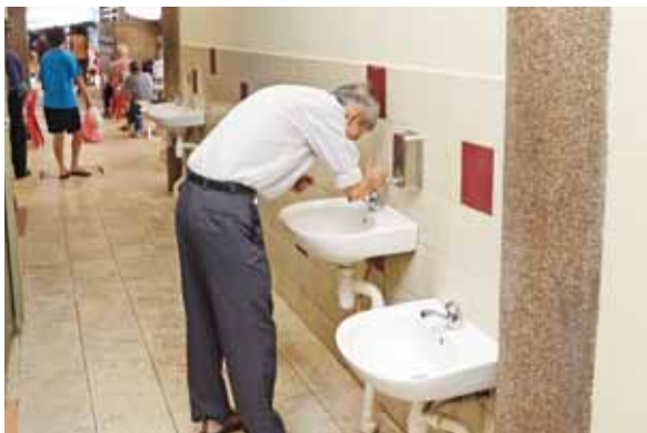
Inside the blocks, you'll find new washbasins, new urinals, new tiling, new plumbing. It's been much more than "Redecoration".
