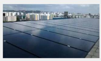
In 2021, we participated in the sixth batch of the SolarNova programme, where 250 blocks were fitted with solar panels that harvest solar energy to power lifts, corridors, staircase lightings, and water pumps in the day. Excess energy was then transferred to the national electrical grid. We have also made plans with the relevant agencies to install more solar panels in the latter phase of the programme.
